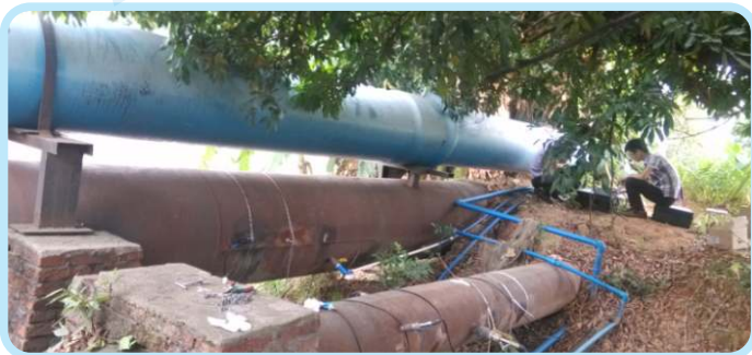
DN800 Water Supply
