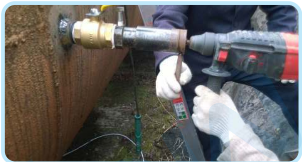
Insertion Transducer Installation
