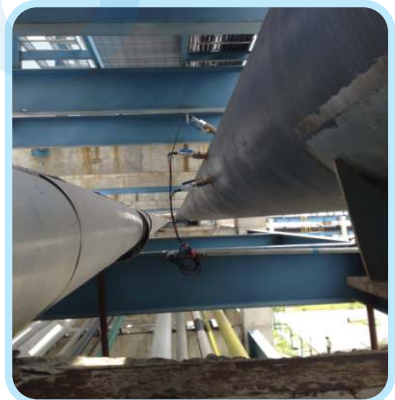
Power Plant Circulation Water
