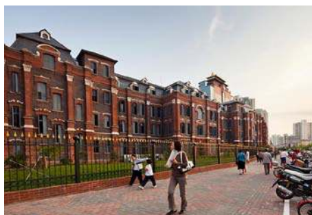
School Dormitory, Residential Building
